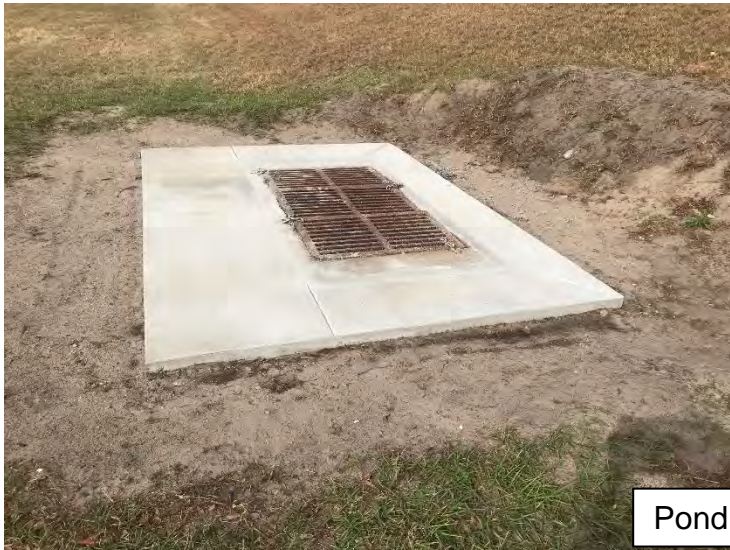
Pond 20, Deepened footing and added rock
