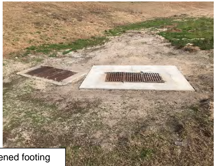
Pond 120, deepened footing and added rock
